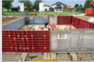
Wall Formwork
