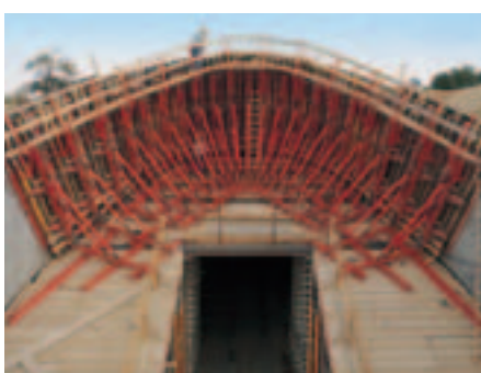
Elliptical-shaped tunnel portal with RUNDFLEX panels and accessories from the VARIO programme. The problem of constantly changing radii and inclination was solved by means of conically-cut filler timbers.
