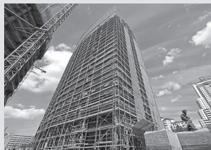
Working scaffolds for facades
