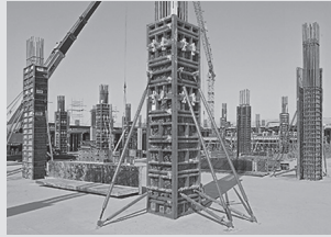
Column formwork
