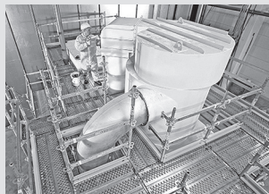
Working scaffolds for industry
