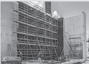
Working scaffolds for construction
