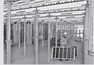
Slab formwork
