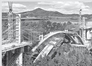
Bridge formwork
