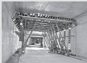
Tunnel formwork
