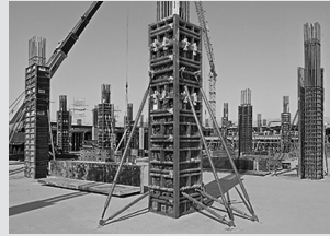
Column formwork
