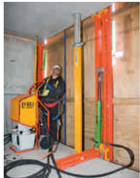
The climbing units are raised with a lifting speed of 1 m/min.
