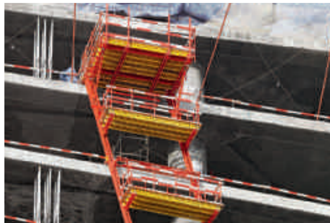
Landing Platforms can also be rail-climbed by means of the mobile RCS Climbing Hydraulics – this additionally minimizes crane usage.
