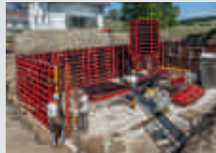
Wall Formwork
