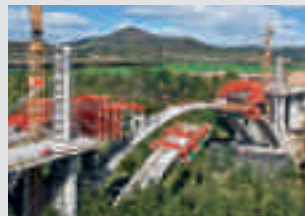
Bridge Formwork
