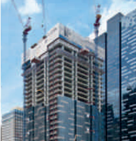
The RCS Climbing Protection Panel in use for the construction of the Asia Square Tower in Singapore. The integrated landing platforms ensure easy transport of materials from floor to floor.
