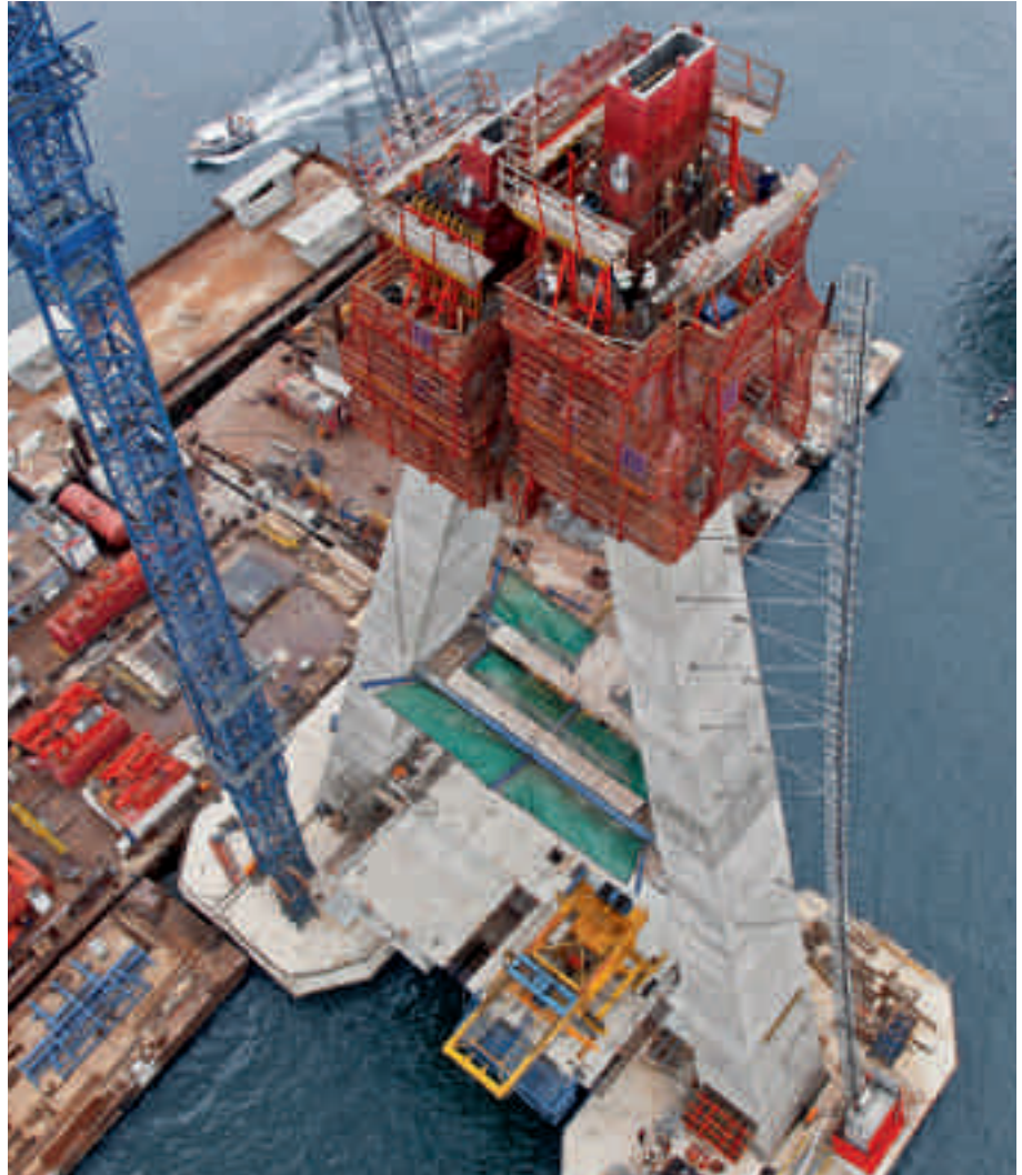
For the pylon of a bridge in Nigeria, PERI combined the ACS and RCS systems. Crane-independent working ensures rapid construction progress in spite of the continuously changing pylon inclinations.
