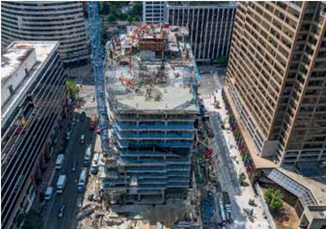
The PERI ACS Core 400 self-climbing formwork shortened the cycle times for the construction of this 31-storey high-rise building.
