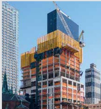
2015 555 Tenth Avenue Residential and Office Complex, New York, United States (LPS)
