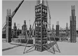
Column Formwork
