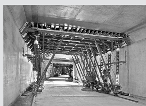
Tunnel Formwork
