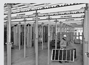
Slab Formwork
