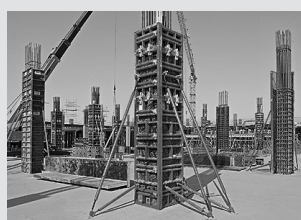
Column Formwork
