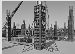
Column Formwork
