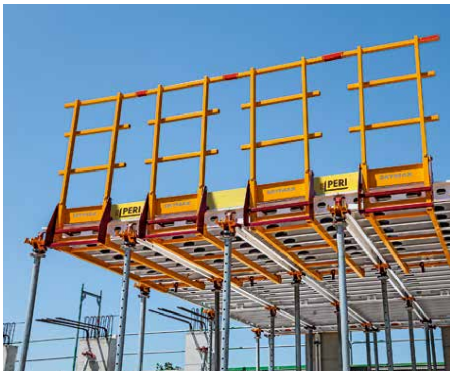
The guardrail unit ensures the safety of personnel and is easy to assemble. You can walk on the SKYMAX system as soon as the anti-fall protection has been assembled.
