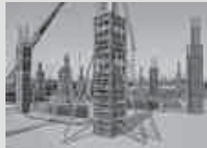
Column Formwork
