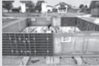
Wall Formwork
